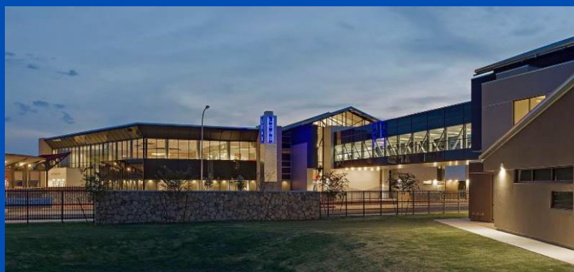
Las Cruces High School Renovations
